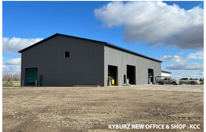
KYBURZ NEW OFFICE & SHOP . KCC
