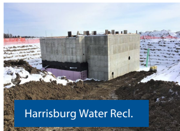
Harrisburg Water Reclamation Facility
