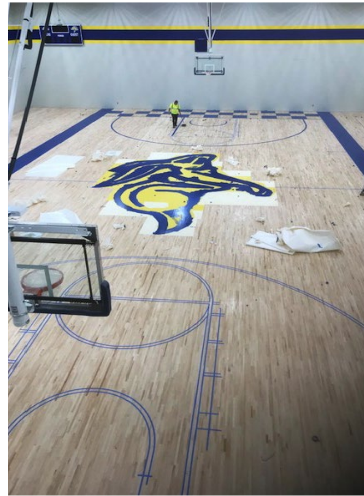
SDSU Stanley J. Marshall Center: SJM is nearing completion, with a completion date of October 29th. The crew had everything painted by October 8th and then two finish coats on top. Commissioning will begin on October 8th. We will have a two week flush out period and this is when the final touches take place. On the exterior, site concrete is ongoing and landscaping has begun. Black dirt has been placed as well and we are waiting for some trees to be placed in the coming weeks.
