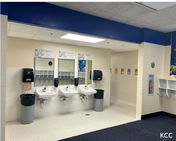
Lincoln Elementary Restroom Renovations
