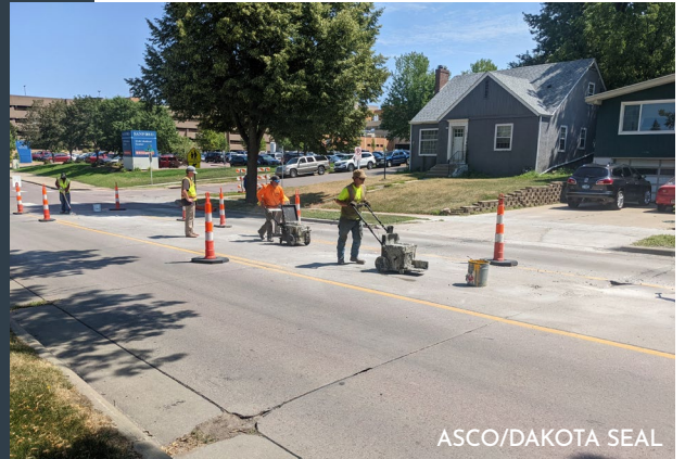
TechCrete Application . 18th Street
