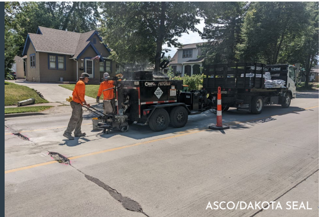
TechCrete Application . 18th Street
