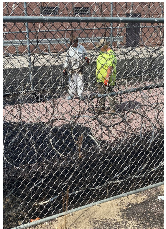
Kudos to Joe Schnellbach and Garrett Berens! They are shooting oil on the slope stabilization rock at the South Dakota State Penitentiary in Sioux Falls. These two have done the majority of this entire project all the way around the Jameson Annex together, going back to 2019. Very labor intensive and meticulous work.
