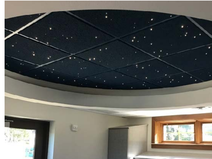
Sanford Ava's House - Each star is an individual fiber-optic cables installed in the blue ceiling tile to create a starry night ceiling.
