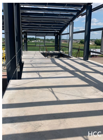
LG Everist Nine Mile Update: The PEMB panels are being skinned onto the Batch Plant at 37 feet high. The Raeco concrete crew has completed the placement at the batch plant mezzanine, and now MEP services are working on the second-floor mezzanine.
