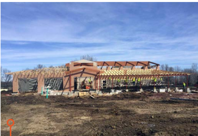
Valley Springs Rest Area . Valley Springs, SD: James McMahon said they are playing in 3 feet of mud at the site, but gluelams are all set, and decking is starting this week. Interstate weigh-in-motion system will start next week as well as grading for the welcome center ramps.
