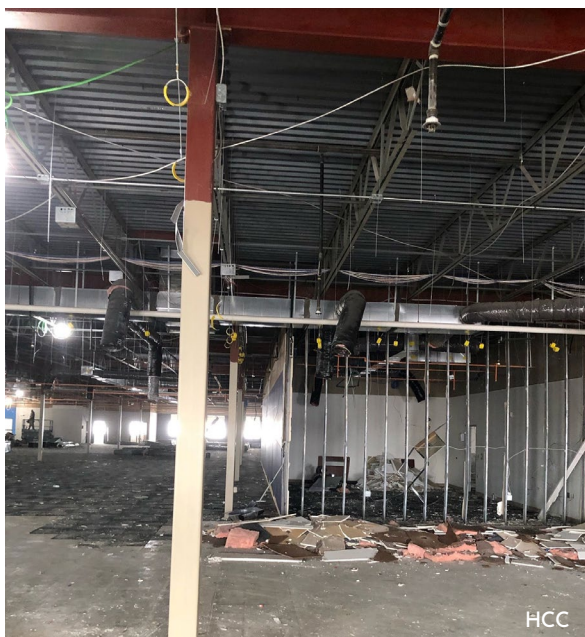
First PREMIER Bank Ops Center (former eSurance Building)
