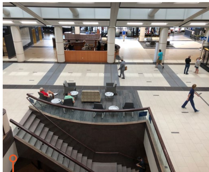
Sanford In-House - Locken Lobby Tile Work
