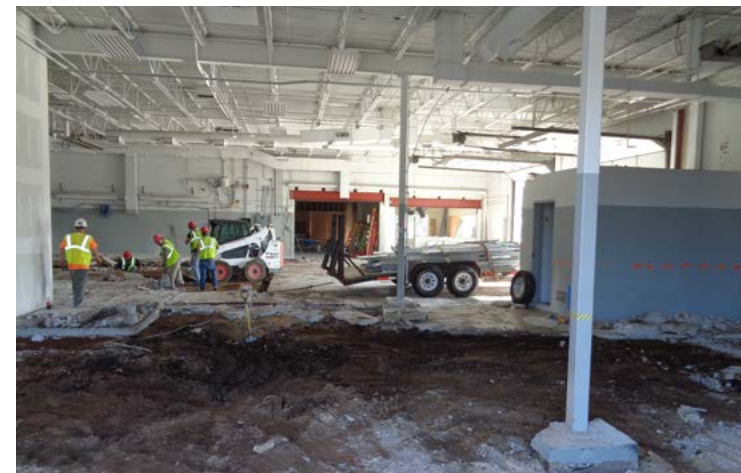
Graham Auto Volvo Demolition - Sioux Falls, SD
