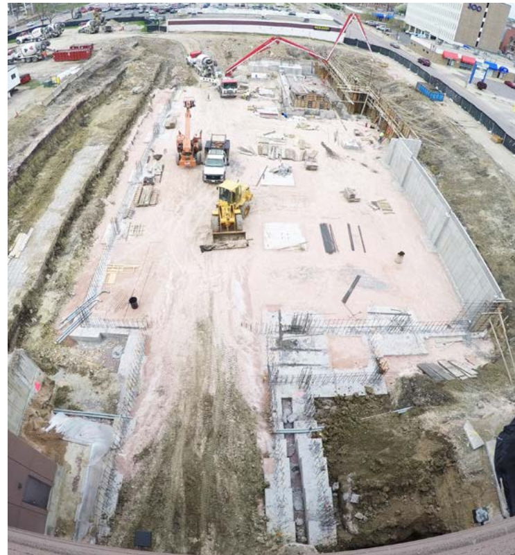
City Administration Building - Sioux Falls, SD
