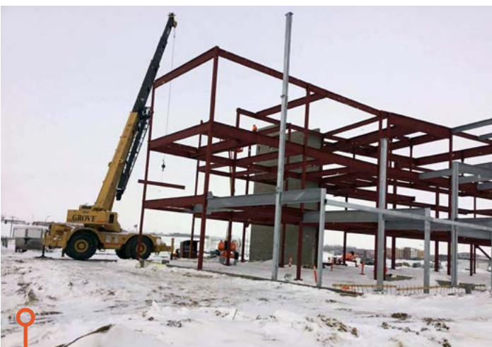
Great Shots . Sioux Falls, SD: The steel crew is about 85% complete with the structural steel. Core floor will be installed in a few days and then the crew will start detailing. The crew is hoping to start decking next week as well.
